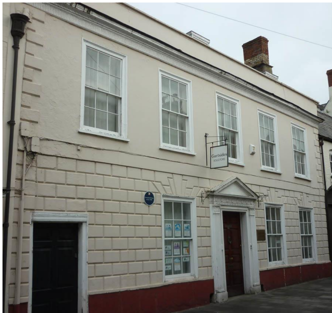
Rother House, 11 Nevill Street (Abergavenny Street Survey)
