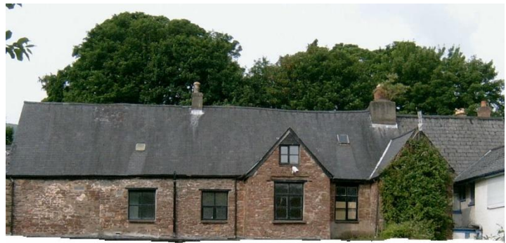
THIS BACK VIEW OF THE GUNTER HOUSE WAS ORIGINALLY THE FRONT.
